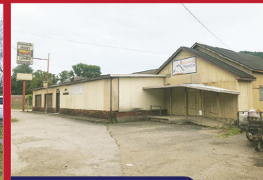
Commercial Building with Fenced Lot
