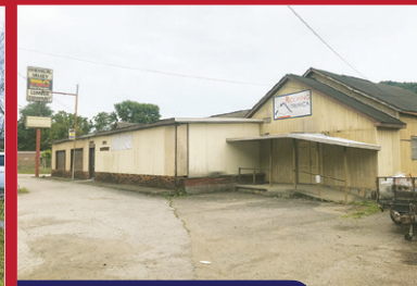
Commercial Building with Fenced Lot
